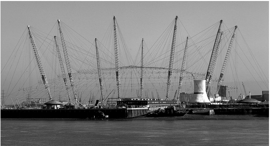
3.23 The Millennium Dome. Cable net before the textile covering was put on.
